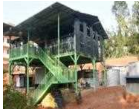
1 MLD STP at Kozhikode medical College
